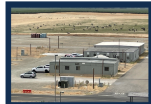
FABS Inspection Trailer Located at the southeast corner of Bellevue Road and Swainson Hawk Lane
